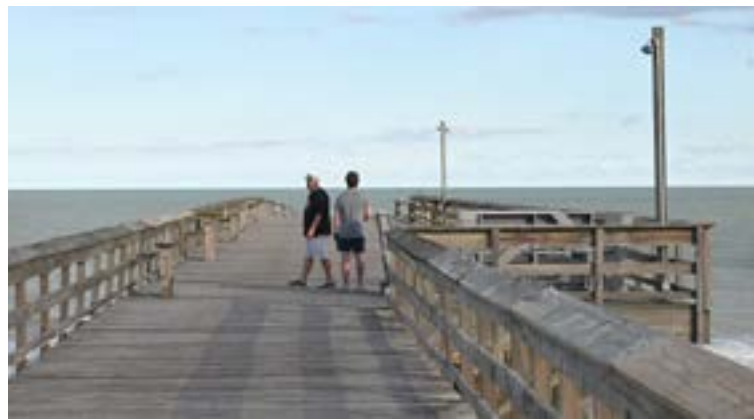
Owners inspect the shortened pier after Hurricane Ian. At top, broken pilings at the end of the pier. The replacement will be the fourth pier to occupy the site on Pawleys Island.
